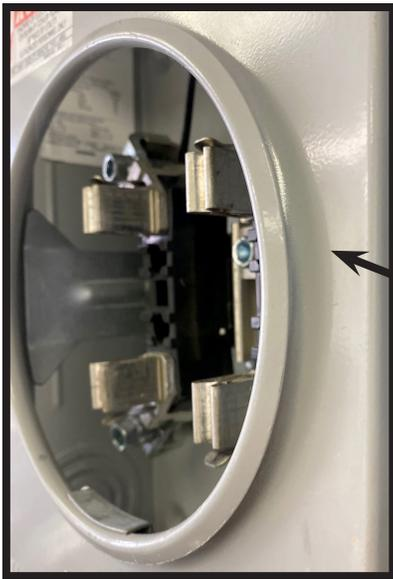
**Ring Style Meter Without Locking/Sealing Ring**
