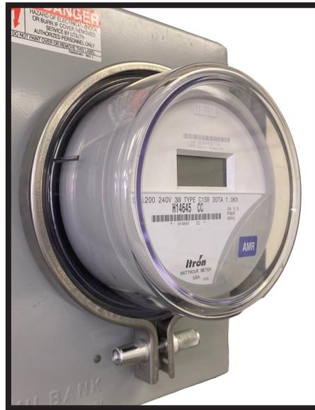
**Ring Style Meter With Locking/Sealing Ring**
