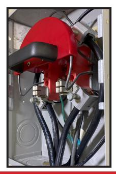
The AE Products Hot Jaw Safety Cover is a cost effective safety product for electrical workers if power disconnect is not an option. This non-conductive design allow work in the lower part of the meter can while blocking the upper jaw blades.
